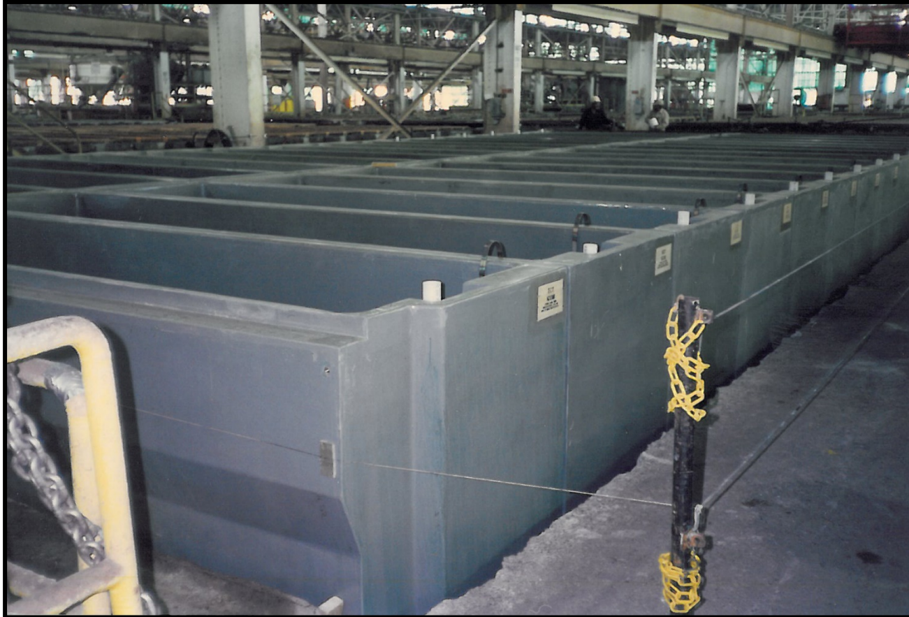
Metals Refining – Electrolytic Cells
